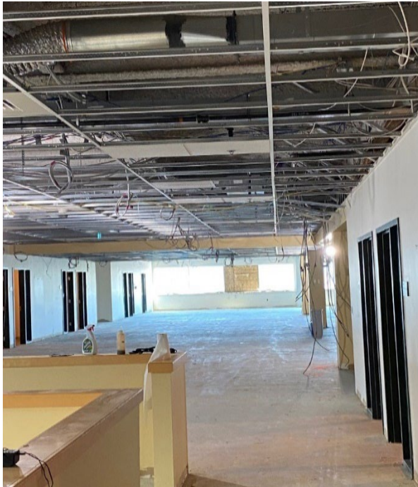
MWRA Office Consolidation - Chelsea Facility
