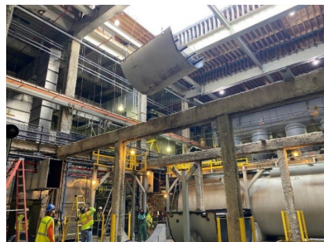
Construction at Nut Island
