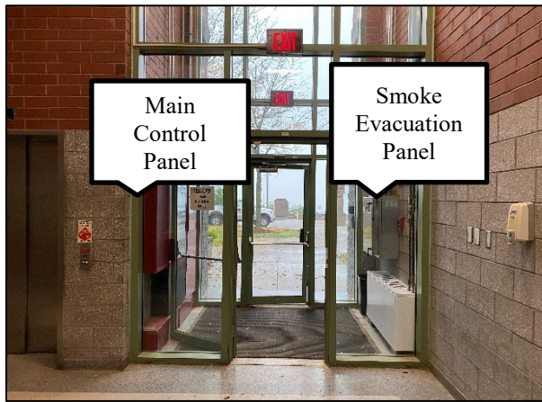
Vestibule at Main Entrance (Fire Command Center)
