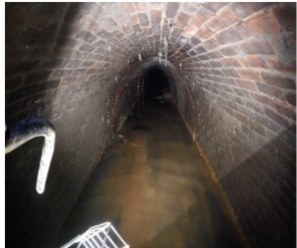
Chelsea 008 CSO Outfall Pipe Replacement
