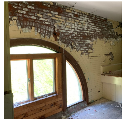
Figure 4: Peeling Paint
