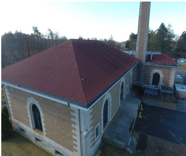
Gillis Pump Station Roof Replacement
