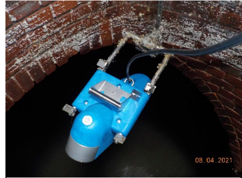
New Wastewater Meter in Sewer
